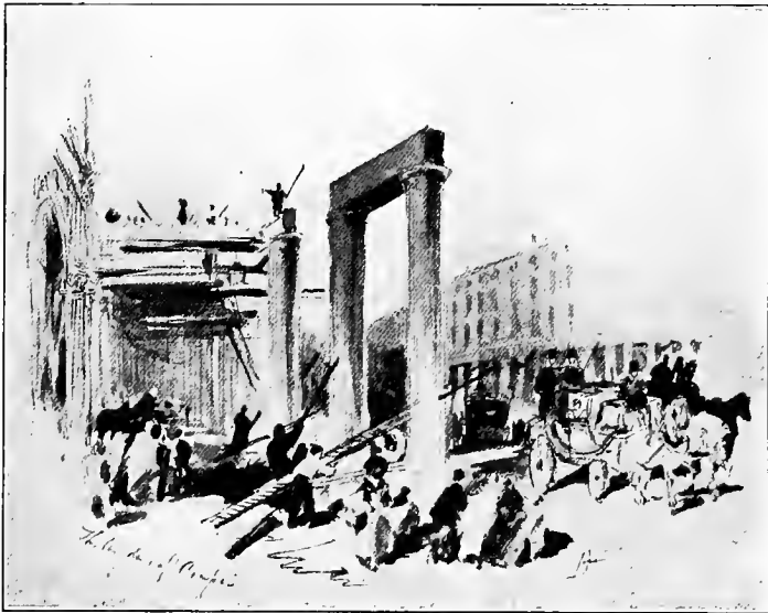
The removal of the Quadrant Colonnade.
